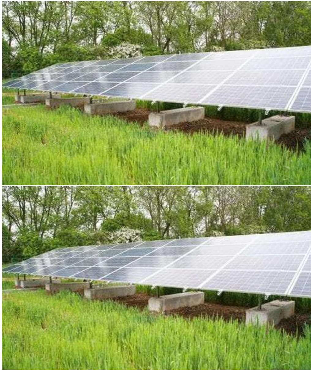
Plate 4.4 Panels on Concrete Feet
