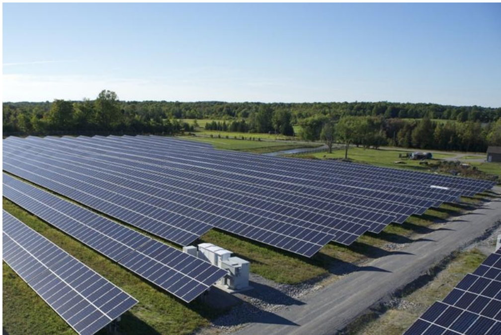
Plate 4.2 Typical Fixed Panels (with Conversion Unit/Inverter)
