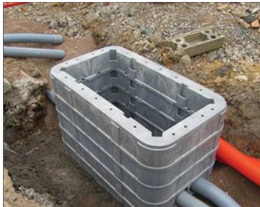
Plate 4.12 Fibre Chambers (construction and external appearance)
