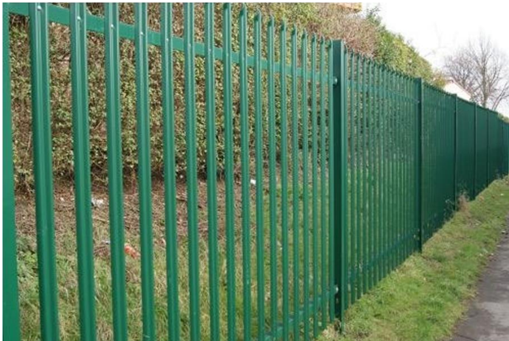
Plate 4.14 Typical Palisade Fencing
