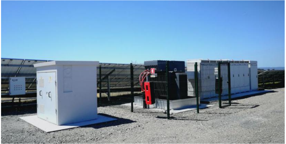
Plate 4.5 Typical Conversion Unit (independent equipment)
